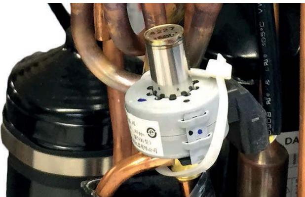
The valve consists of an electrical operator and a valve body with internal variable size orifice. When operating, the PCB will send pulses of voltage to the electrical operator. The operator will then magnetically move the position of the metering orifice pin to vary the flow of refrigerant.
