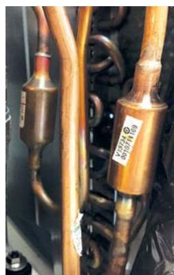
The system has debris-catching strainers that protect internal system components from contaminants. The strainer is a permanent part that is not typically replaced.
