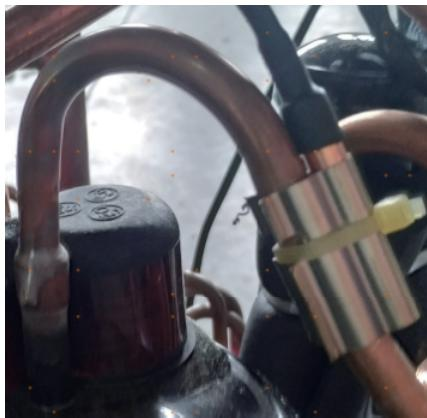
The Discharge Sensor is a negative coefficient thermistor that senses the temperature of the compressor hot gas. The PCB will make inverter speed changes in response to input from this device.
