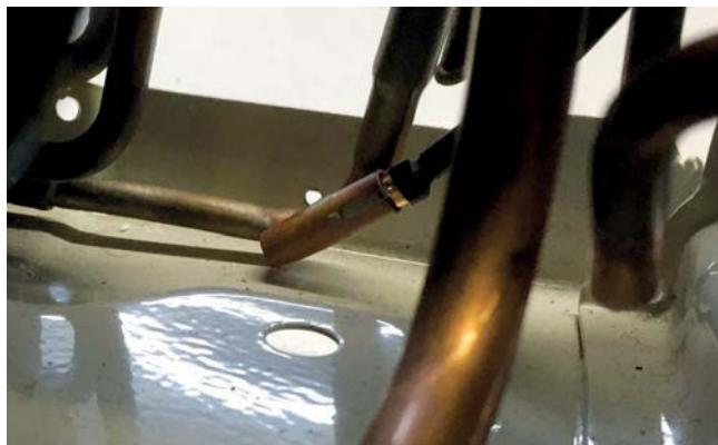
The Defrost Temperature Sensor is a negative coefficient thermistor that will change resistance in response to outdoor coil temperature changes. The Main Control Board monitors the temperature of the outdoor coil to determine when a defrost cycle is necessary. The sensor also monitors outdoor coil temperature during defrost cycles to determine termination conditions.
