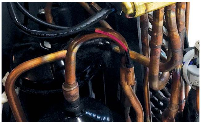
The Suction Line Temperature Sensor is a negative coefficient thermistor that senses the temperature of the suction line to determine EEV orifice size, maintaining in an attempt to maintain proper operating superheat.
