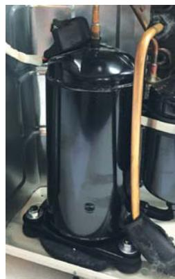
The compressor is a three phase DC inverter-driven rotary. The compressor is capable of variable speed operation. The operating frequency will be determined by the difference between set point and room emperature.
