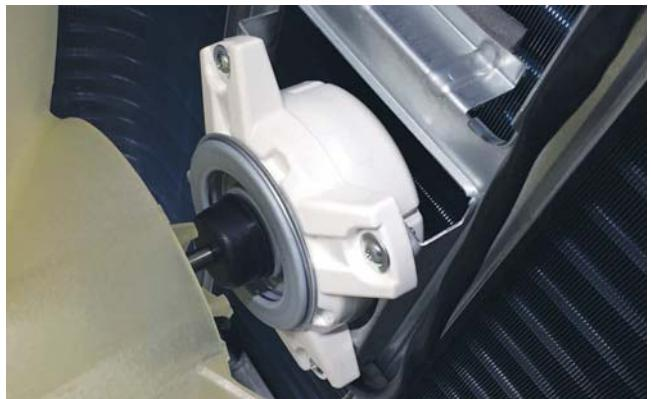
The fan motor is a variable speed DC motor, The required motor speed is calculated by the Main Control Board. The motor is electrically connected to the PCB via CN21 (09k and 12k), or CN22 (18k and 24k).
