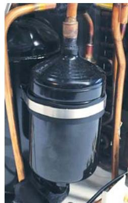
The Accumulator is located in the suction line at the entrance to the compressor. The accumulator helps prevent liquid refrigerant from entering the compressor.
