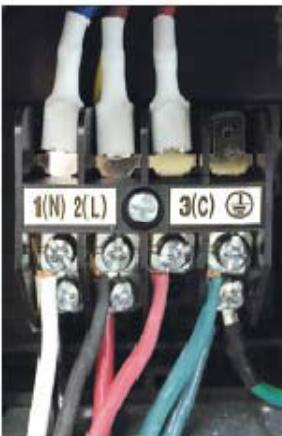
The terminal block receives electrical power from the outdoor unit. Terminals 1 and 2 are connected to terminals 1 and 2 of the outdoor unit. This wiring supplies power to the indoor unit.
