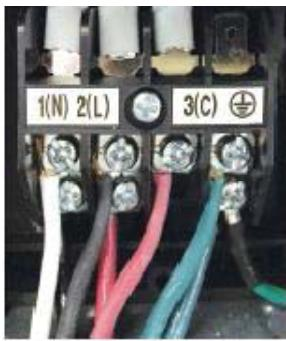
The 18K and 24K units are 208/230 volt single phase. The 9K and 12K units are 120 volt. All models use terminals 1 and 2 as incoming power wiring. Number 3 is the communication terminal and the 4th terminal is the ground connection. Be sure to match this wiring with the indoor unit terminals.
