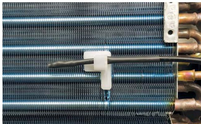
The Ambient Sensor is a negative coefficient thermistor that will decrease in resistance with increases in room air temperature. The sensor is located on a clip mounted to the surface of the indoor coil.
