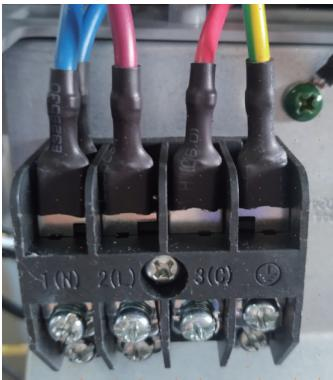
The outdoor unit is powered by 208/230 volt single phase electricity connected at the terminal block.
