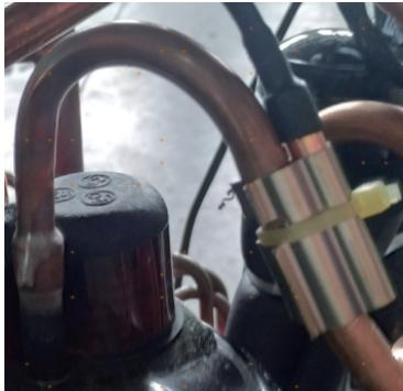
The Discharge Temperature Sensor is a negative coefficient thermistor that senses the temperature of the compressor hot gas. The PCB monitors the temperature of the compressor hot gas and will make inverter speed changes in response to input from this device.
