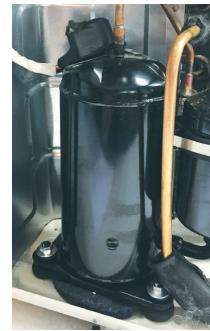
The compressor is a three phase DC inverter driven rotary type, capable of variable speed operation. The compressor operating frequency will be determined by the temperature difference between set point and room temperature.
