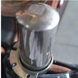
The metering device is an electronic expansion valve. The valve consists of an electrical operator and a valve body with internal variable size orifice. When operating, the PCB will send pulses of voltage to the electrical operator. The operator will then magnetically move the position of the metering orifice pin to vary refrigerant flow.
