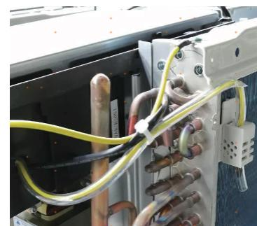
The Defrost Temperature Sensor B is same as the Defrost Temperature Sensor A. The system chooses the lowest of the two temperature values.
