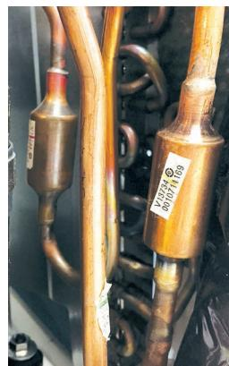
The system has debris-catching strainers that protect internal system components from contaminants in the refrigerant. The strainer is a permanent part that is not typically replaced.
