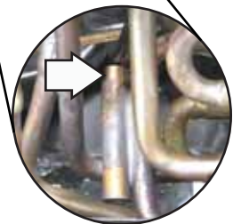
Outdoor Coil Thermistor
