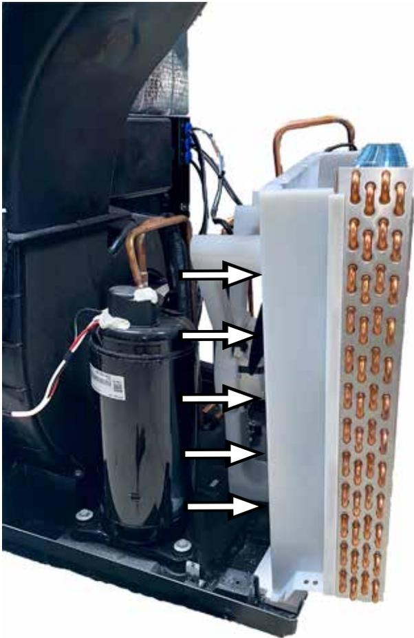
7. Remove the fan assembly from the outdoor coil by pulling up on the assembly.
