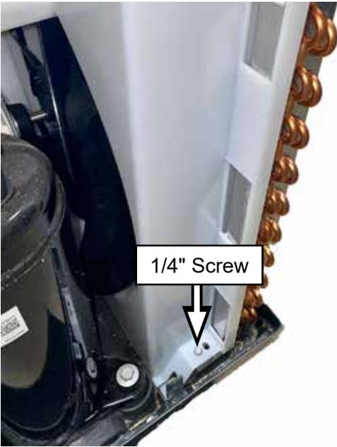
6. Near the compressor, pull the outdoor coil and fan assembly slightly out. This will allow the fan assembly to slide up without hitting the outlet duct.
