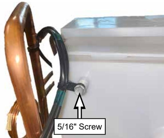
3. Clip zip tie holding the thermistor harness to the tubing. **NOTE:** Install a new zip tie to the tubing and harness after replacing the thermistor.
